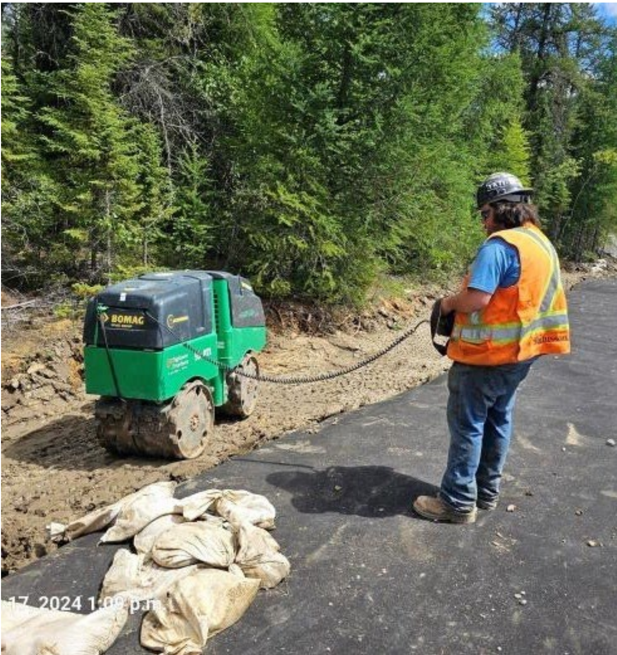
Anchor Trench Installation with Clay Compaction
