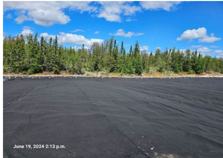
4. Seamed geotextile with hot guns
