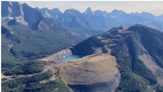
An aerial view of Tent Mountain in southwestern Alberta, which was the site of an open-pit coal mine that was active decades ago but has since been abandoned. Montem Resources now aims to use the site for a pumped-hydro energy storage project. (Montem Resources)
